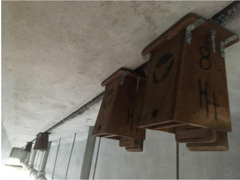
Plate 2.1 Example of alternative microbat boxes secured with anchor bolts into insitu slab (between expansion joint) on a super-T bridge. The microbat boxes are re-enforced with galvanised steel brackets securing the lid to the side.
