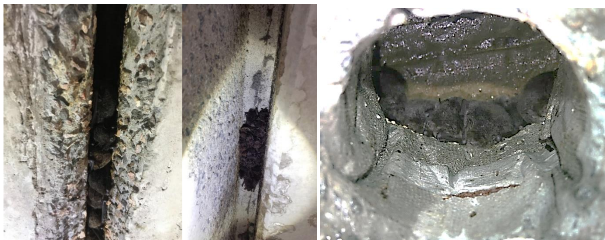
Plate 2.2 Examples of concrete texturing on bridge and culvert structures to create/enhance microbat roost habitat values.
